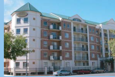
Windsor Apartments, Adelaide, SA, Value: $848,000, No of Bricks: 350,000
