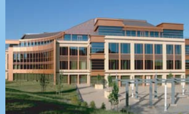
Sydney Avenue, Canberra Act, Value: $0.5 million, No of Panels: 101, Feature: Yellow Sandstone Sand Blasted
