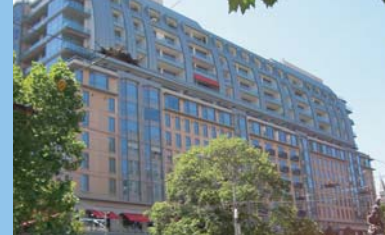
Westin Hotel, Melbourne Vic, Value: $2.0 million, No of Panels: 331, Features: 280 Curved and Polished
