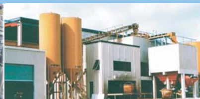
Computerised Concrete Batching Plant
