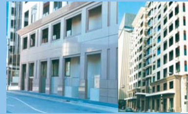
Australian Taxation Office, Waymouth Street Adelaide, Value: $1.3 million, No of Panels: 321, Feature: Heritage Style Podium
